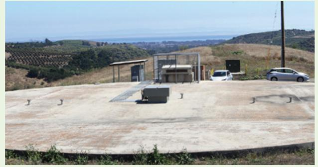
*Reservoir aeration treatment was installed at Ellwood Reservoir to treat and remove disinfection byproducts*
