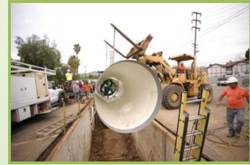
Riverside Public Utilities installed an in-line hydroelectric generator in a 48-inch pipe that utilizes the flow of water to generate electricity. The spherical turbine generates between 2 and 7 kilowatts of energy on a continuous basis, depending on the velocity of water through the pipe, and poses no threat to fish or wildlife.
