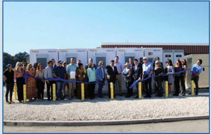
The District celebrated its 80th anniversary with a ribbon cutting for the new Battery Storage Project at the CDMWTP.
