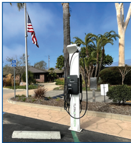
Mounted EV chargers and installed related electrical conduits in-house, saving $45K.
